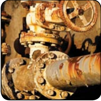
Flange Corrosion
