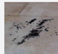
Holes in the roof of an AST
